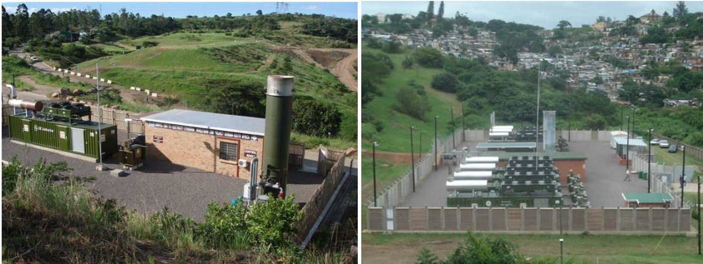
**Figure 1:** The Mariannahill 1MW (left) and Bisasar Road 6,5MW (right) landfill gas to electricity CDM projects which were CDM-registered and commissioned in 2006 and 2009 respectively.
