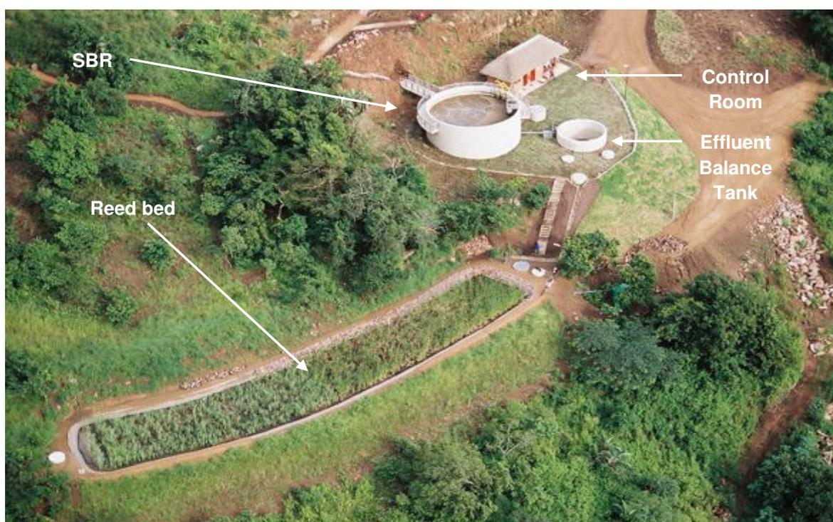
Figure 1. The Mariannahill Leachate Treatment Plant, a 50m<sup>3</sup>/day ‘prototype’ for the new 200m<sup>3</sup>/day Buffelsdraai leachate treatment plant.
