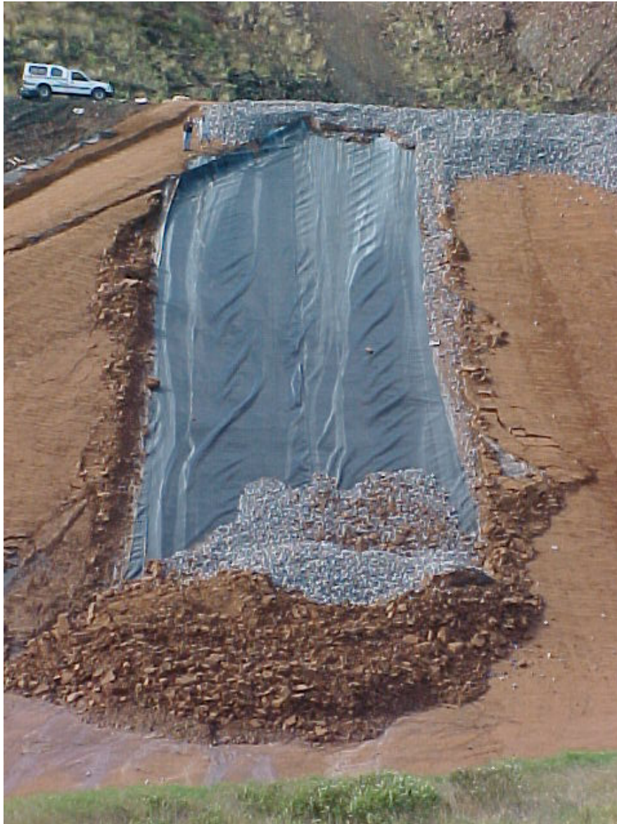
Figure 4. Bisasar Road Landfill Site Randles 2d : View of Slope after First Slide
