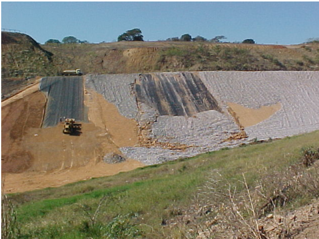
Figure 5. Bisasar Road Landfill Site Randles 2d : View of Slope after Second Slide
